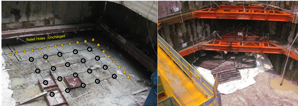
Figure 5-2: Schematic View of Blasting Design (left) and Blasting Area After Charging Stage (right)
